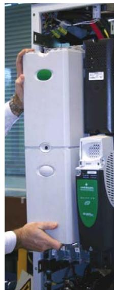
The SPMD drive in this picture is capable of controlling 350A (200kW induction motor, typical) and yet is extremely manageable. The picture shows it being installed in a 400mm wide cubicle.
