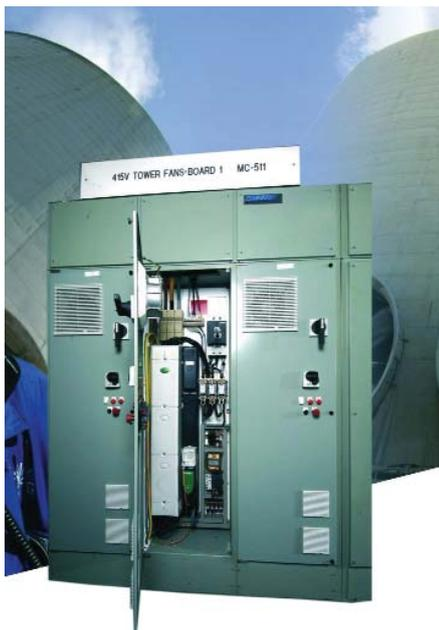
In this example, from the power generation sector, the requirement was to find a 132kW drive that would fit inside an industry standard motor control cubicle, to increase reliability and maximise generating efficiency. The SPMA was a unique solution.
